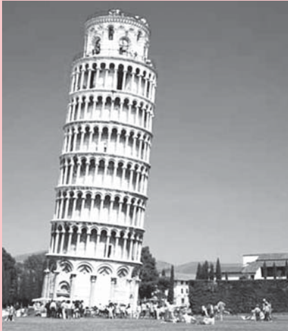
Leaning Tower of Pisa
