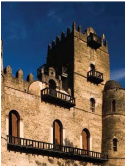
Figure 7.21 Part of Fasilidas's palace in Gonder. Are the balconies in equilibrium?
